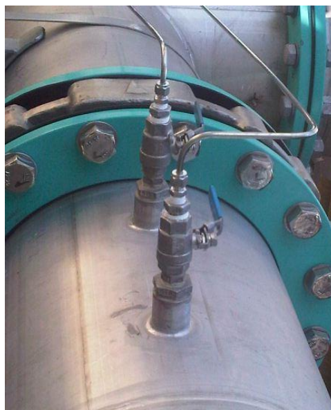
Figure 7 - Ball valve assembly
